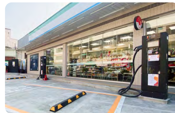
Convenience store charging station
